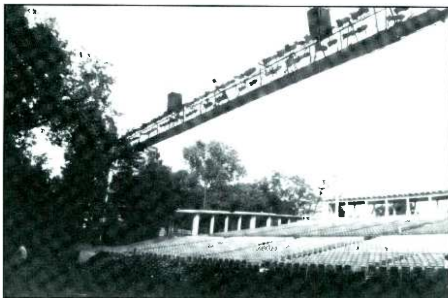
Figure 2. The speaker system is Apogee 3X3-IIs flown from cable above the audience.
