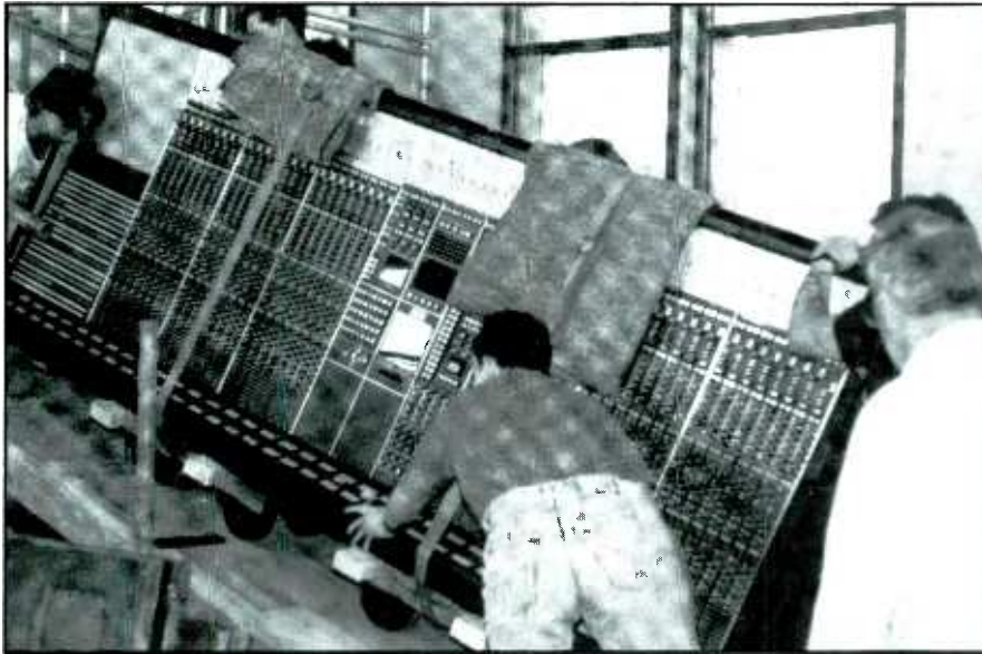
Figure 3. The decision to scale down the studio's size resulted in an even better facility. Here, the new SSL is being moved in.
