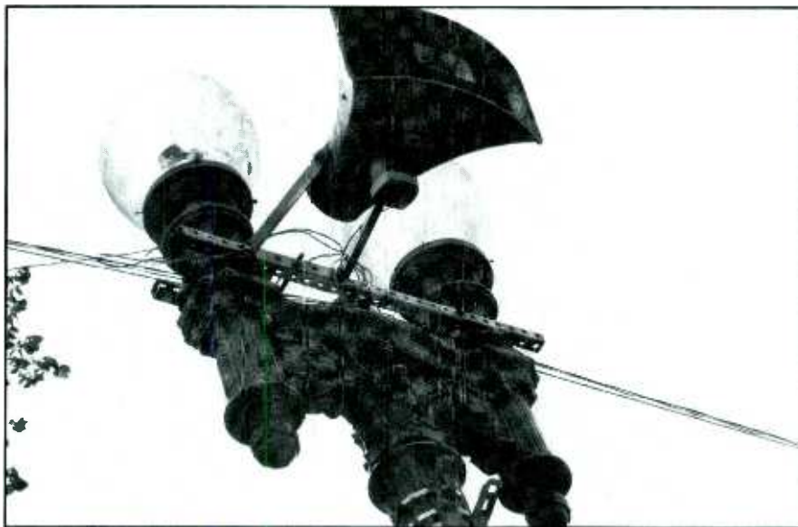
Figure 4. A close-up of the Unistrut fastening system for the D.C. lamp posts.
