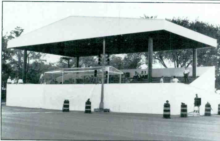
Figure 9. Workmen putting the final touches on the Presidential reviewing stand. Note the bulletproof glass enclosure for President Bush.
